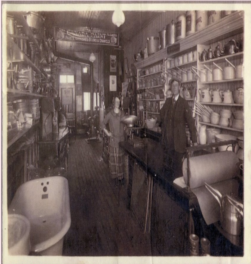
Lloyd Tetlock and assistant. Tetlock Plumbing and Heating, 126 Bridge Street, c. 1935.
